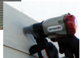
Fiber Cement Siding to Steel
