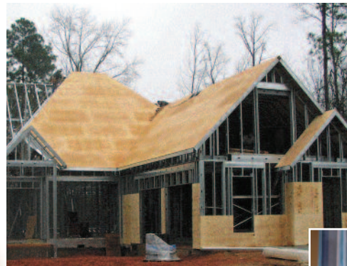
Plywood/OSB to Steel
