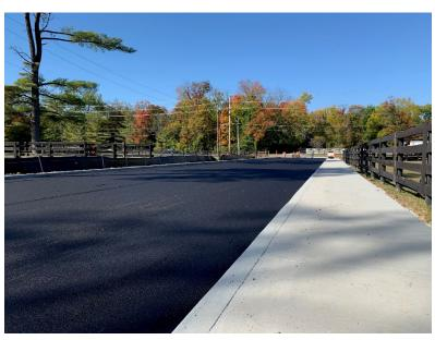
The south driveway is finally complete! The driveway was widened to allow for two-way traffic, and a sidewalk was added for safety.
