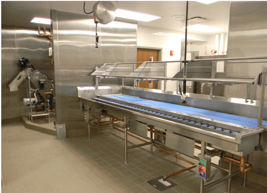
In the dishroom, staff take advantage of a pulper and the scrapping and extracting area of the dishroom as well as the tray conveyor leading to the dish machine. Photo by Libby Shoop, marketing manager, C&T Design and Equipment
