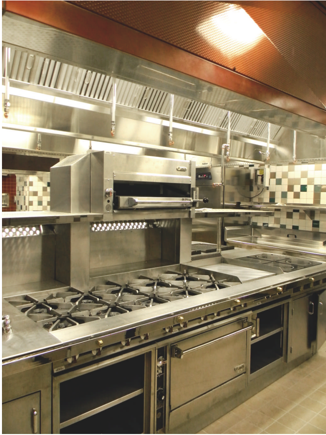
Clockwise from left: In the cooking suite of the servery area are a range, mounted broiler, griddle and induction support production.
